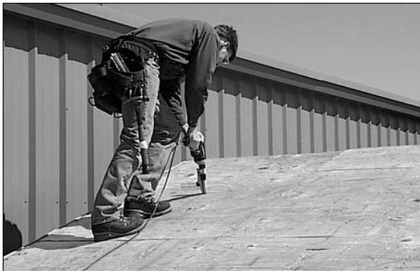
**3.** Have the sheathing refastened using either 8d ring-shank nails or #8 screws 2 inches long (see listing of auto-feed screw guns). The nails or screws should be installed between the existing fasteners and at a spacing of not more than 6 inches between the old and new fasteners. A smaller spacing (4 to 5 inches) is recommended if the ring-shank nails are used. Also, if
