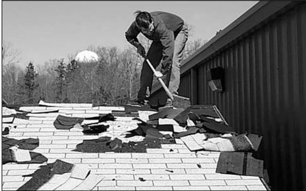
**2.** Have the roof sheathing inspected for damage or decay. Replace any weak material with sheathing rated for your truss or rafter spacing (16 or 24 inch).
